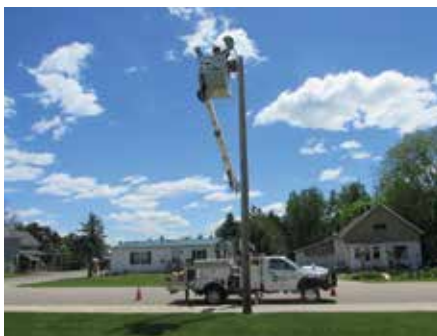
Lineman John Bestul works to replace the street lights to energy efficient LED bulbs.
