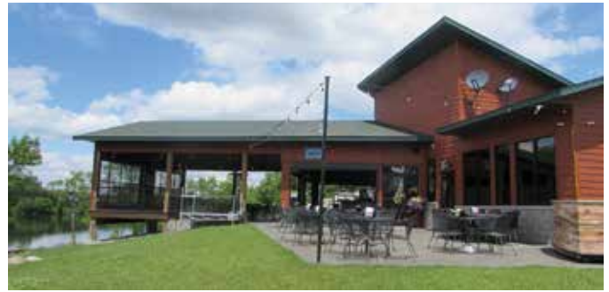
Bullhead's Bar's deck doubles as a stage for concerts.
